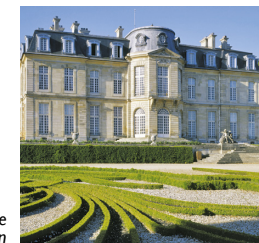
The façade facing the garden
